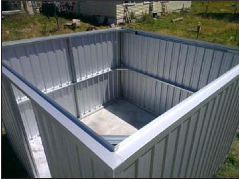
*Figure 3. Shoebox flashing.*
